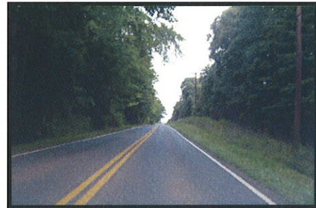
Cel-River Rd. Facing West Near Site
